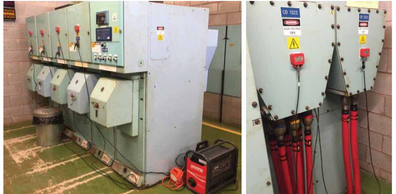
Short-term Monitoring of 11 kV Switchgear with HVPD Kronos® Portable Monitor
