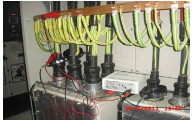
Testing on the 33 kV Cable Joints
