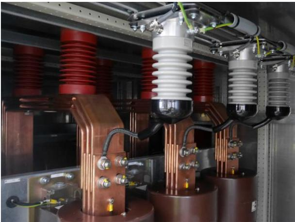
**Figure 3 Example of 15 kV, 500 pF HVCCs installation on a 15 kV, 45 MW generator.**
