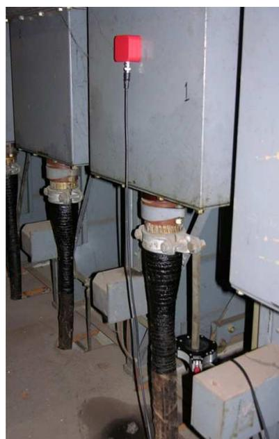
**Figure 9: Photo of TEV Sensor Attachment to Cable Box and HFCT connection to Cable Earth Bar**
