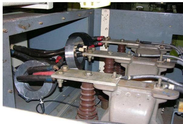
**Figure 15: HFCT Connections on 6.6kV Generator**
