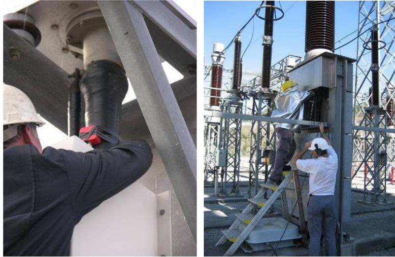
**Figure 1** Sensor attachment to 132kV (left) and 220kV (right) cable sealing ends
