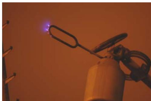
Figure 1. Low Light Photograph of Discharge on Sealing End Arcing Horn
