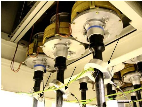
**Fig 2 High frequency current transformers (CT's) around cores of 33kV cable for PD measurement (CT's are arrowed)**
