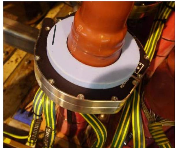
Fig. 5 An installed TB-3 sensor
