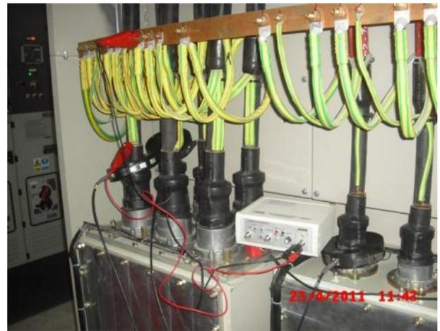
Figure 10 Mapping of the 33 kV network of a metropolitan rail system.
